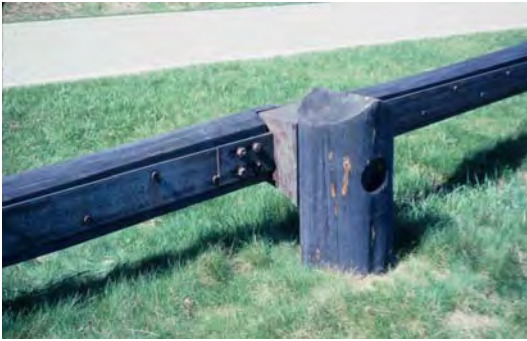
Caption: (Left) Steel-backed timber guardrail on the Blue Ridge Parkway in Virginia. The barrier is crash-tested and approved by the federal government and is available in blocked-out (as shown in a blocked-out design for higher speed roads) post and rail configurations. (Right) The New Mexico DOT uses an adobe-colored coating to help guardrails better blend into the natural and historic landscape of the state. Old Las Vegas Highway, the first alignment of U.S. Route 66 in New Mexico (New Mexico State Scenic Byway). Paul Daniel Marriott
