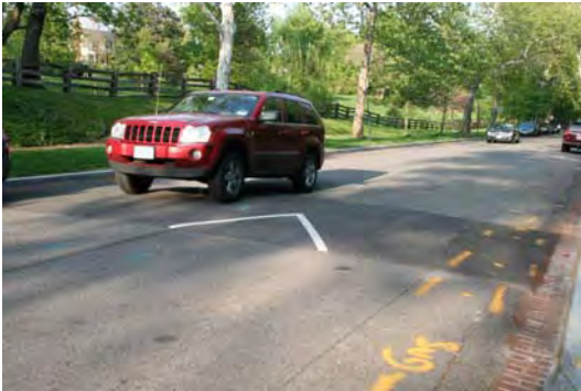
Caption: Speed humps, such as this one in Washington, DC, are the most common form of traffic calming. Paul Daniel Marriott
