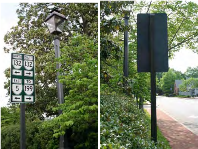
Caption: The City of Williamsburg, Virginia clusters highway information and uses smaller route shields (as allowed by MUTCD) in built up areas and along lower speed roads. The backs of the signs are painted to minimize the visual impact on the landscape. Paul Daniel Marriott
