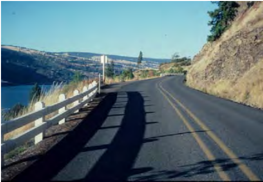
Caption: The Historic Columbia River Highway (National Historic Landmark, National Scenic Byway--All-American Road) pioneered a post and rail wooden barrier in 1915. No longer suitable for safety requirements, the barrier was redesigned as a part of the highways restoration and rehabilitation. The posts are slightly larger, and the rails are now reinforced with galvanized steel. The barrier has been crash-tested and approved for use on appropriate facilities by the federal government. Paul Daniel Marriott
